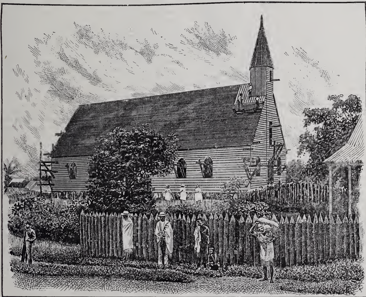
HOVA CHURCH, TAMATAVE, IN COURSE OF ERECTION. NOW IN RUINS.
